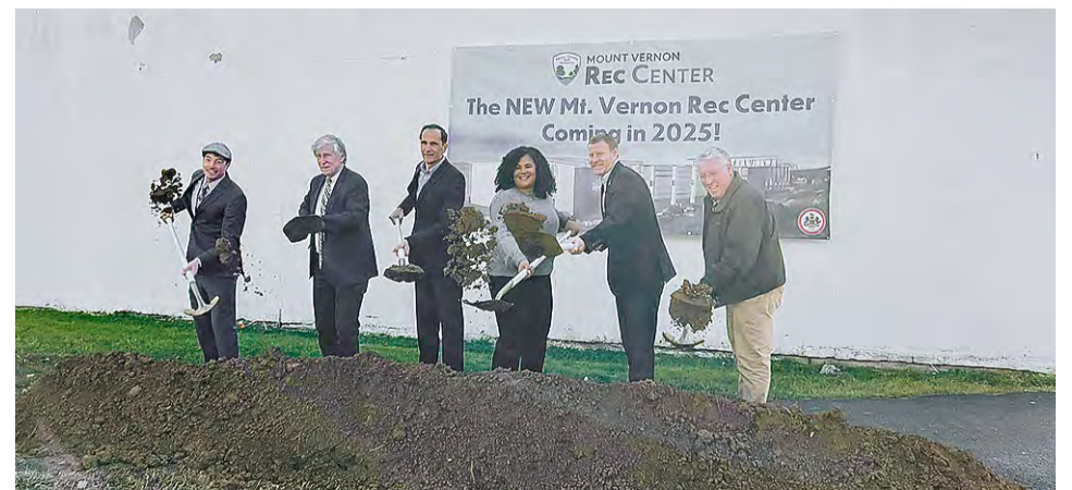
On Jan. 18, officials gathered to break the ground for the renovation of Mount Vernon Recreation center. Although this recreation center will be closed for two years while the work is going on, the new center will grow to 75,000 square feet of recreation space which includes a second ice rink.
